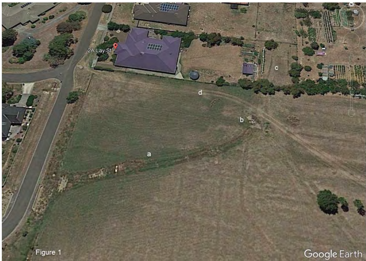
Figure 1. Drainage at 44 Ingliston Drive and 2A Lay Street, Ballan. a). open drain, b). stormwater inlet, c). open drain and underground storm water pipe, d). low area caused by driving cars across wet ground.
