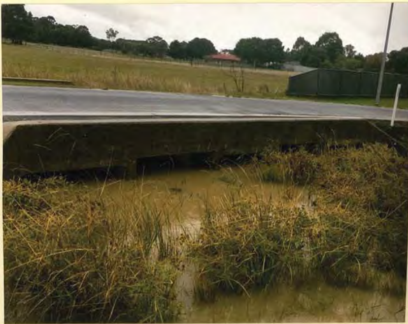
LAY COURT BOX CULVERT LOOKING EAST (WEST SIDE)
