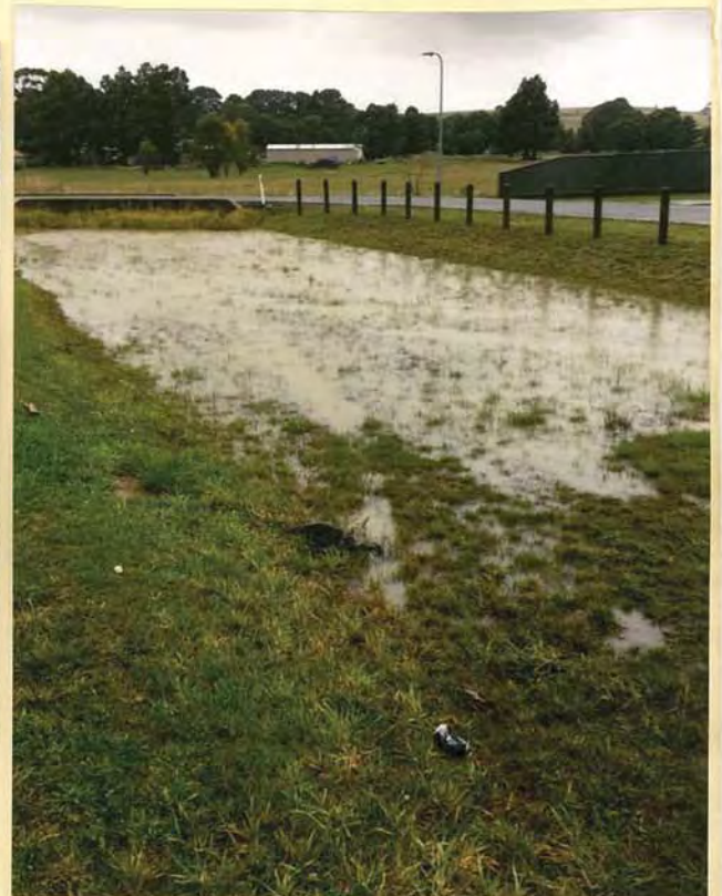
LAY COURT DRAINAGE CHANNEL LOOKING EAST
