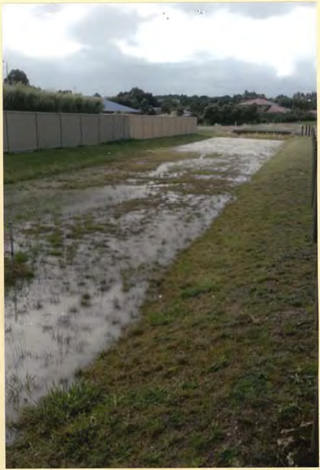
LAY COURT DRAINAGE CHANNEL LOOKING EAST
