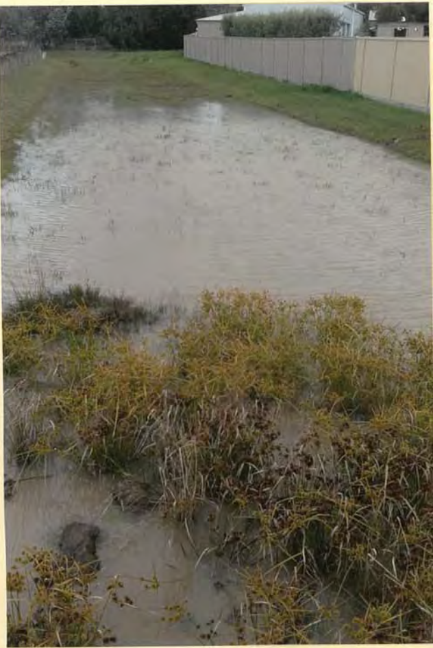
LAY COURT DRAINAGE Channel LOOKING WEST.
