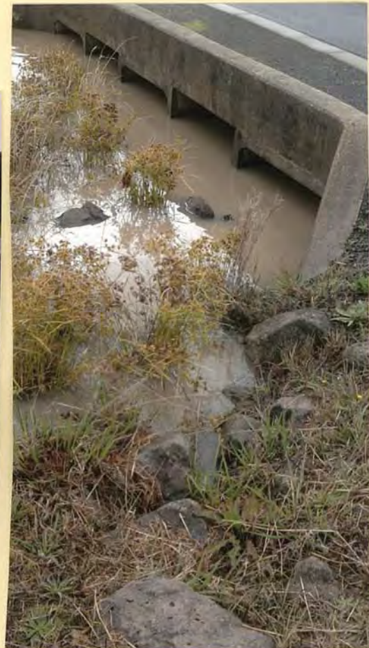
EAST SIDE OF BOX CULVERT
