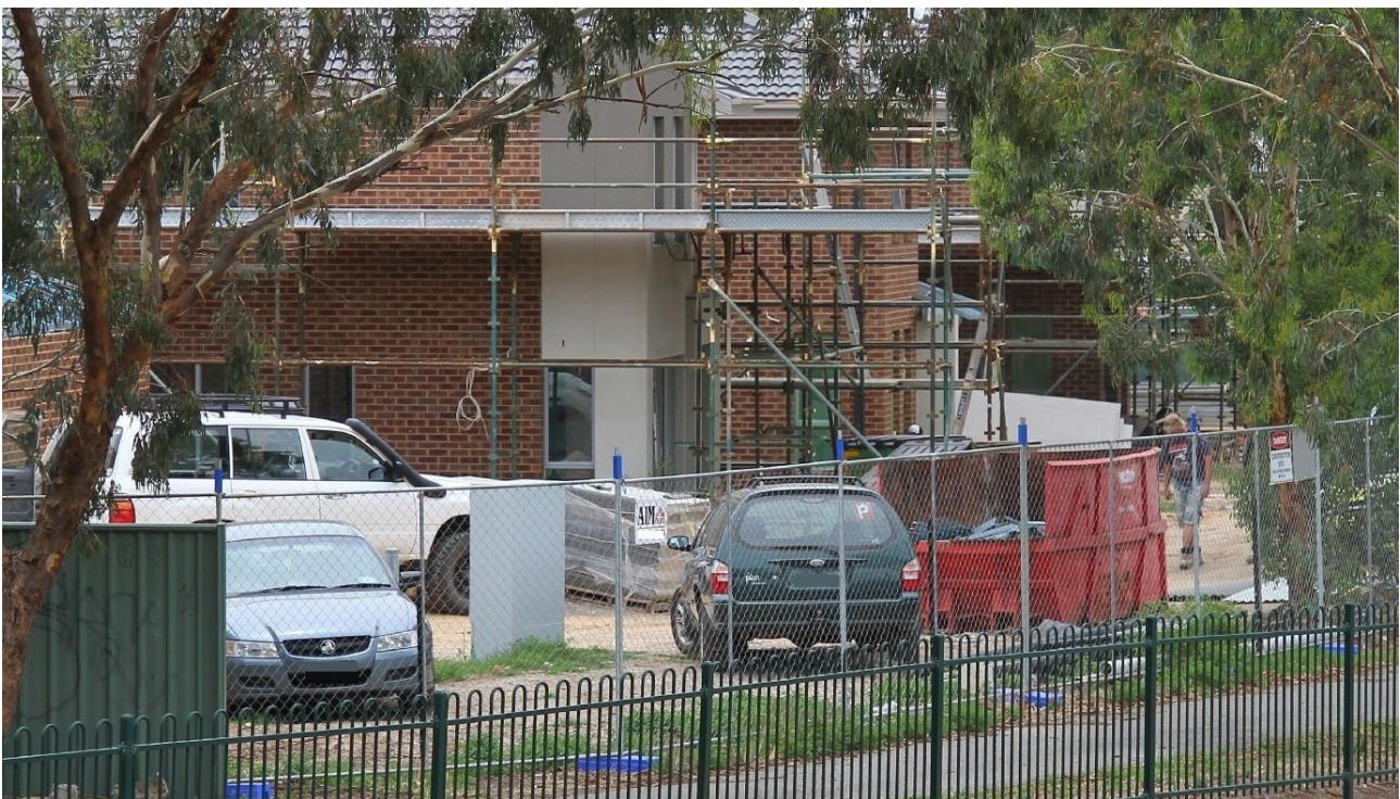
Construction adjacent to a creek in Bendigo
