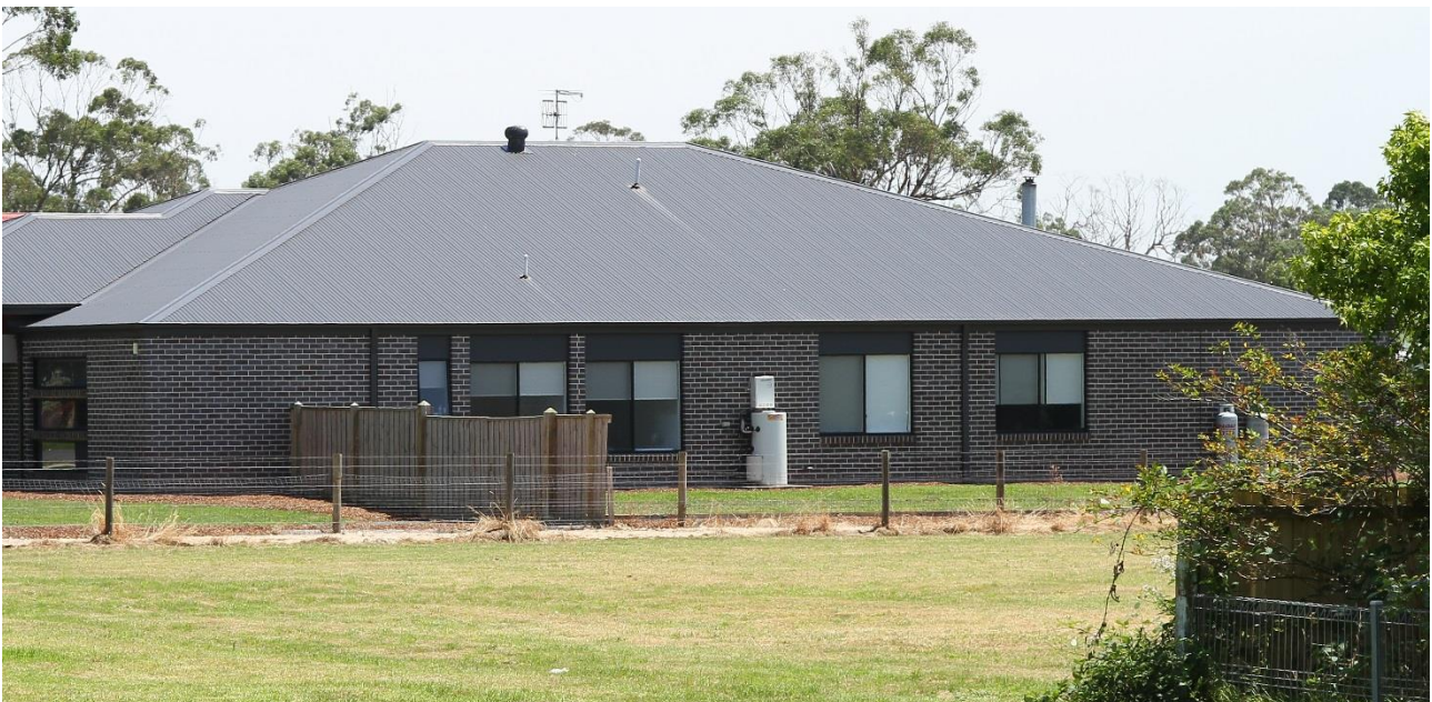
New dwelling on a fill pad Credit: Ian Gauntlett, DELWP
