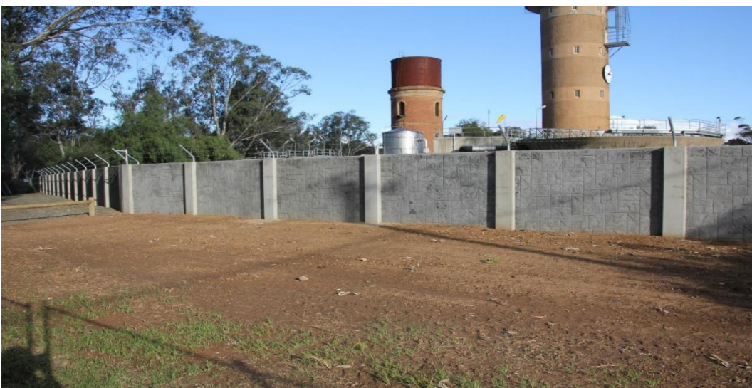
Flood protection levee – Rochester Water Treatment Plant
