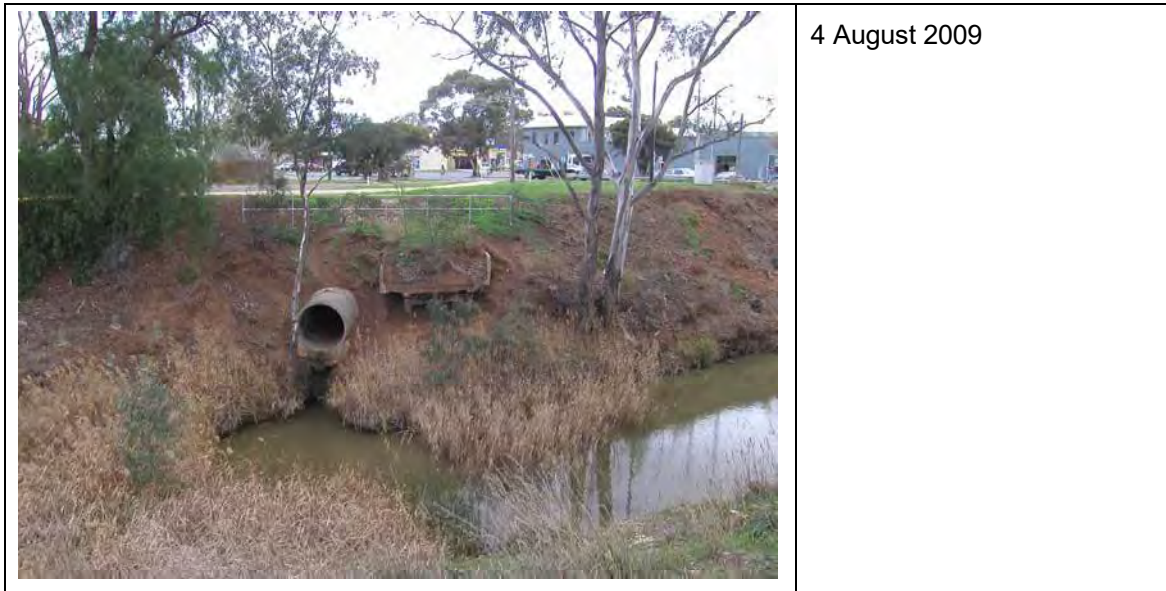
Figure 4-4 Maddingley Park Drain outlet at the Werribee River near Grant St
