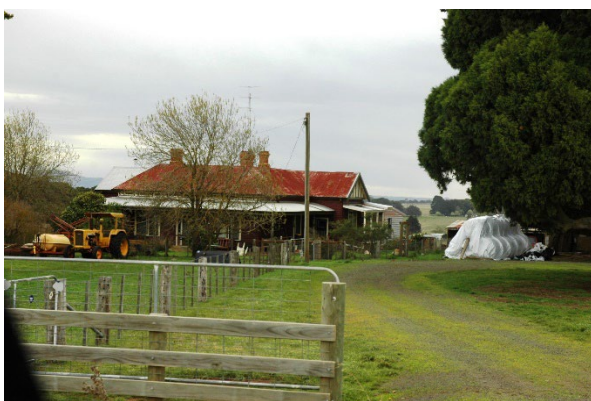
Photo 2: Main entrance showing the main dwelling, 2009.
