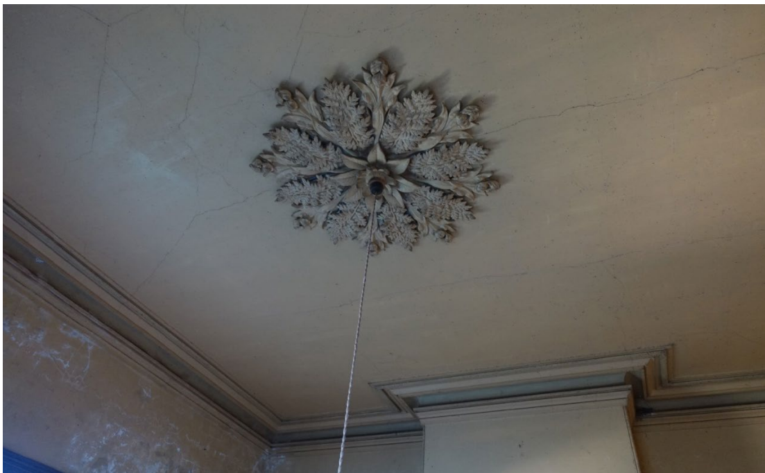
Photo 8: Ceiling of the south-east (front) room, showing the plaster cornice picked out in three colours and the papier mâché ceiling centre, 2025.
