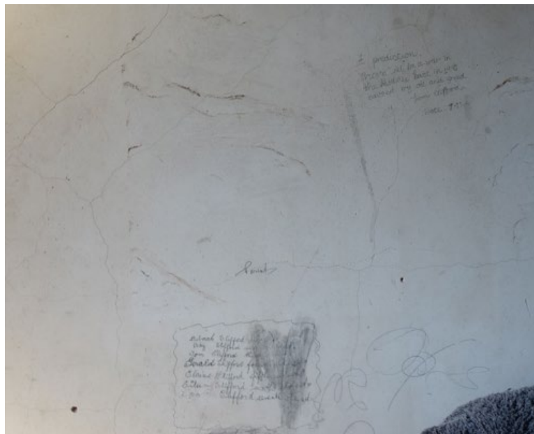
Photo 10: Pencilled graffiti on the east wall, near the window of the first-floor north-central room, 2025.
