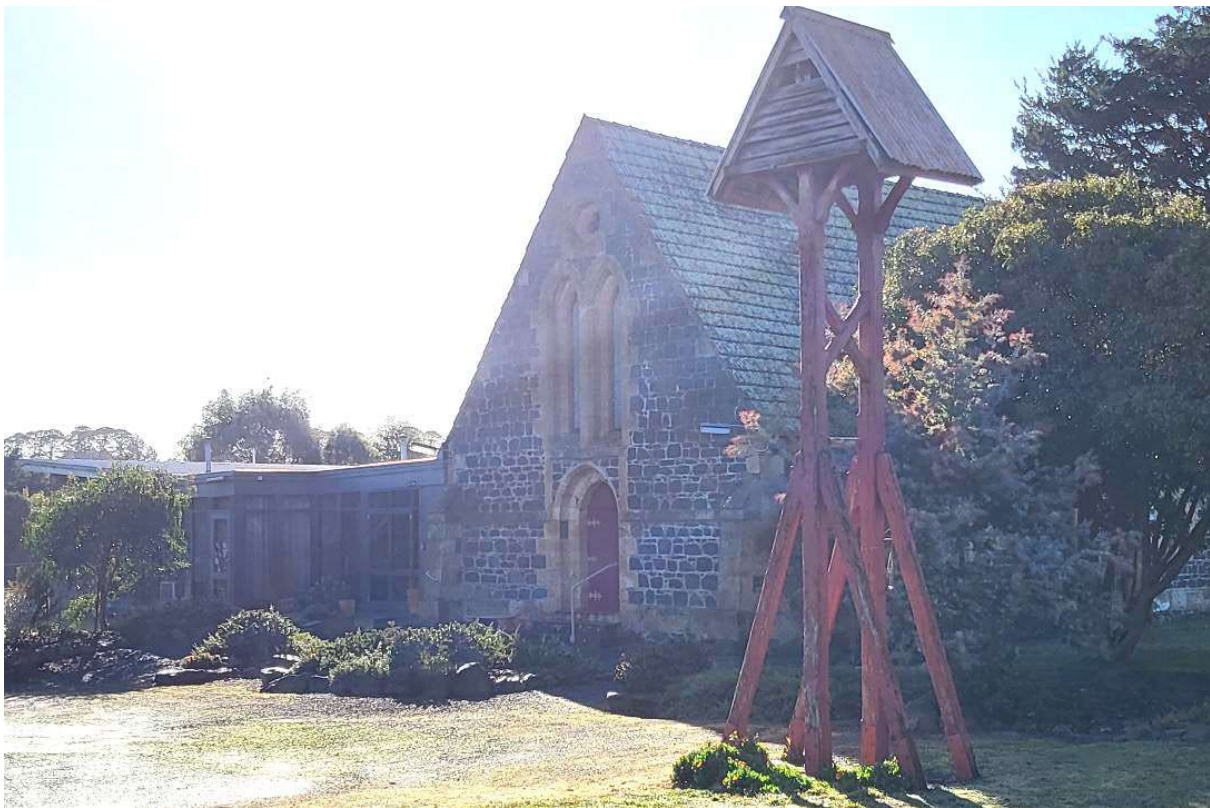
Figure 2 St Johns Anglican Church bell tower
