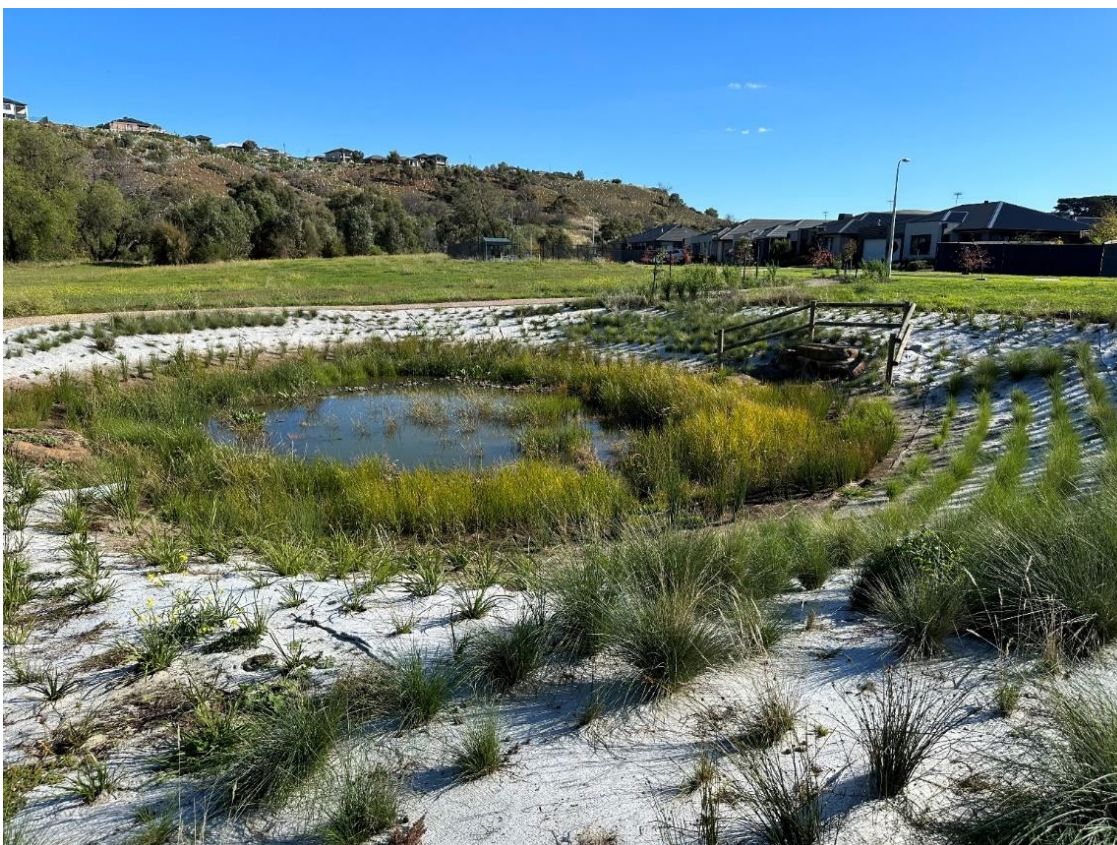
FIGURE 4.9: PHOTO OF EXISTING SEDIMENTATION POND AND BIORETENTION SYSTEM AT RIVER EDGE
