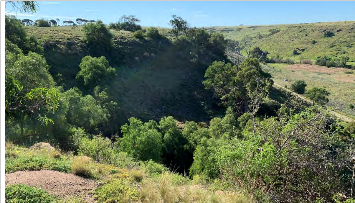
Figure 11 View of eastern scarp near Hopetoun Park Road, looking north, showing very steep slopes with basalt outcrops in the upper part of slope. The floodplain at the base is periodically inundated as part of Melton Reservoir pondage.
