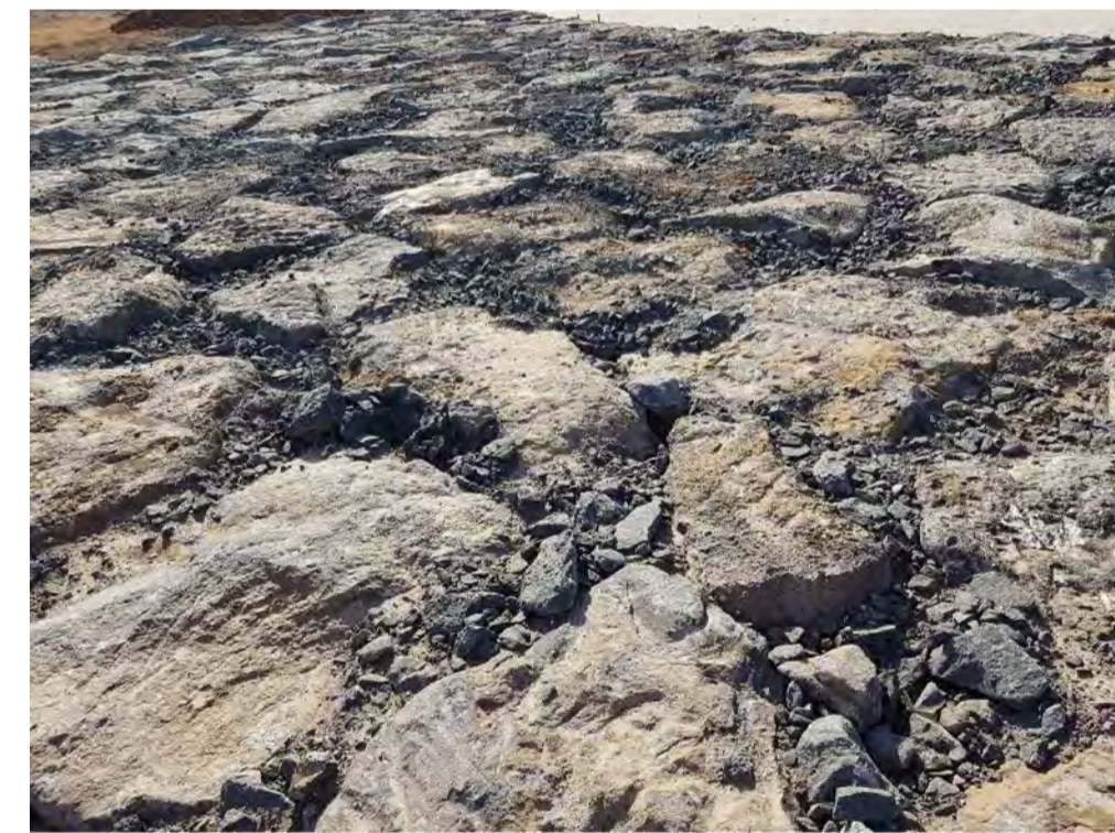
EXAMPLE OF WELL INTERLOCKED ROCKWORK WITH SEALED VOIDS
