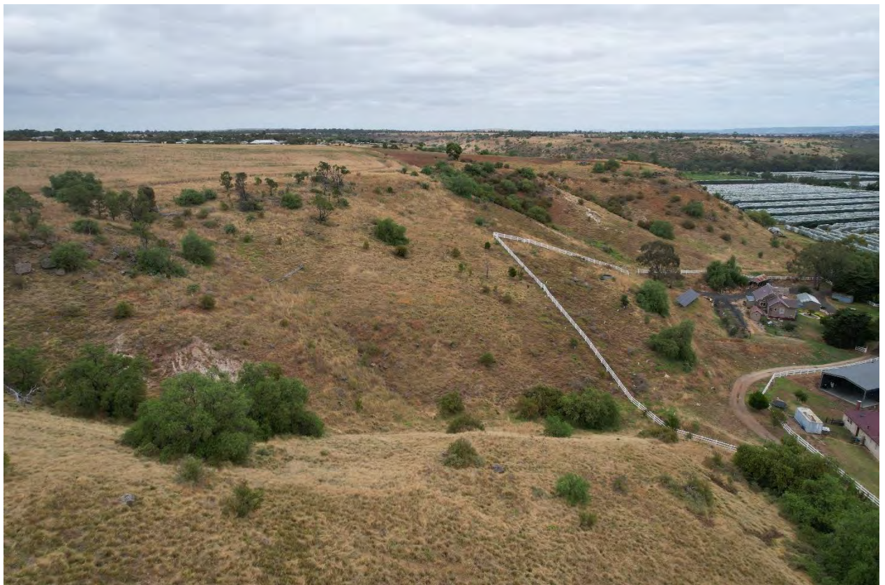
Image 29 – Aerial view to south from north.
