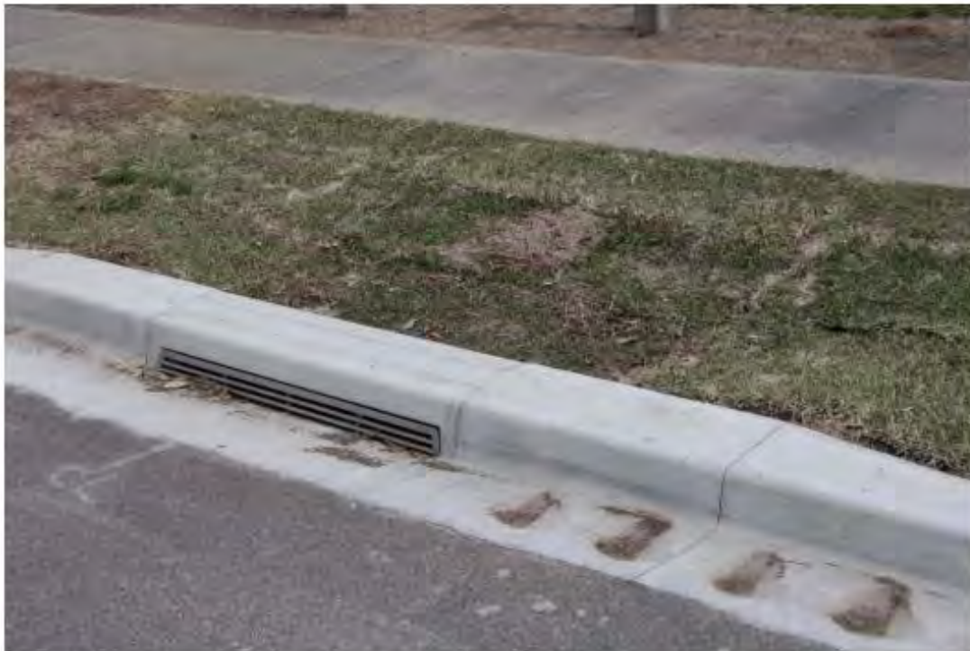
Park Avenue, Doncaster, single barrier kerb installation
