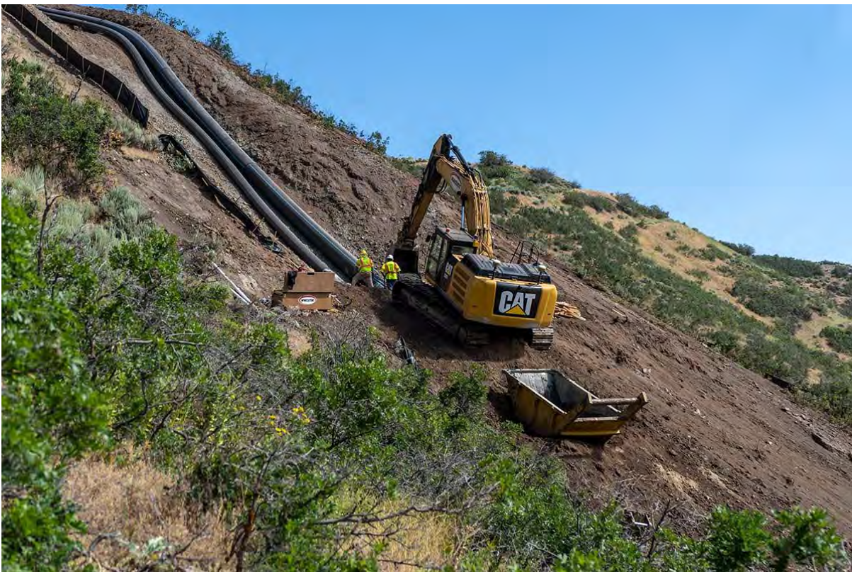
Figure 49. Polyethylene (black) pipe installed on a steep slope (Source: Google Images, 2020)
