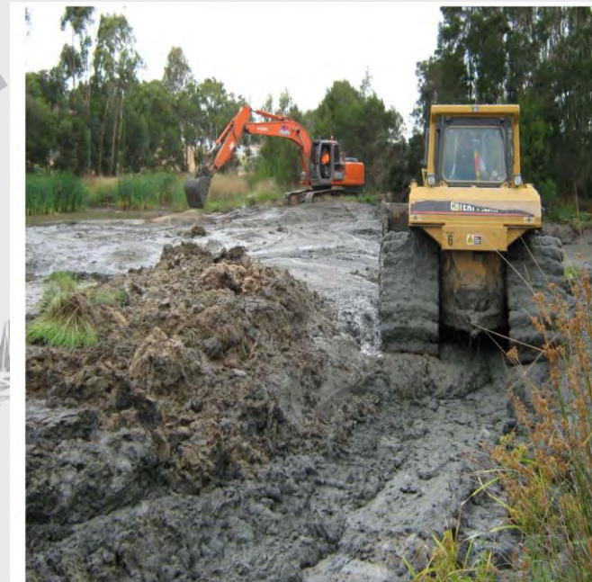
Figure 7: Excavator and swamp dozer on the pond floor removing sediment.
