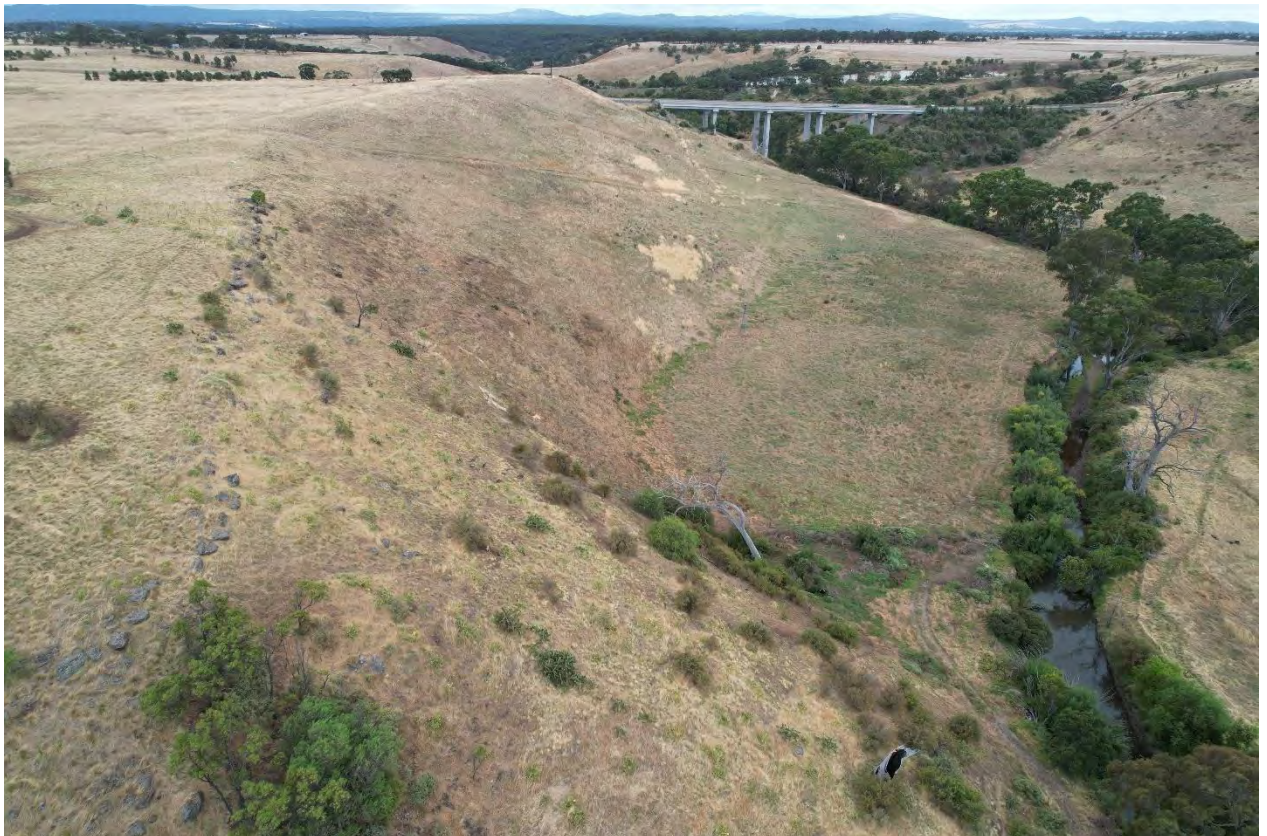
Image 16 – Aerial view towards the north.
