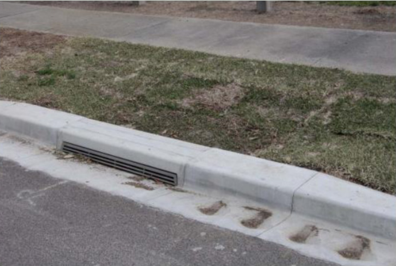
Fig. 7 Example ZAM sediment treatment system
