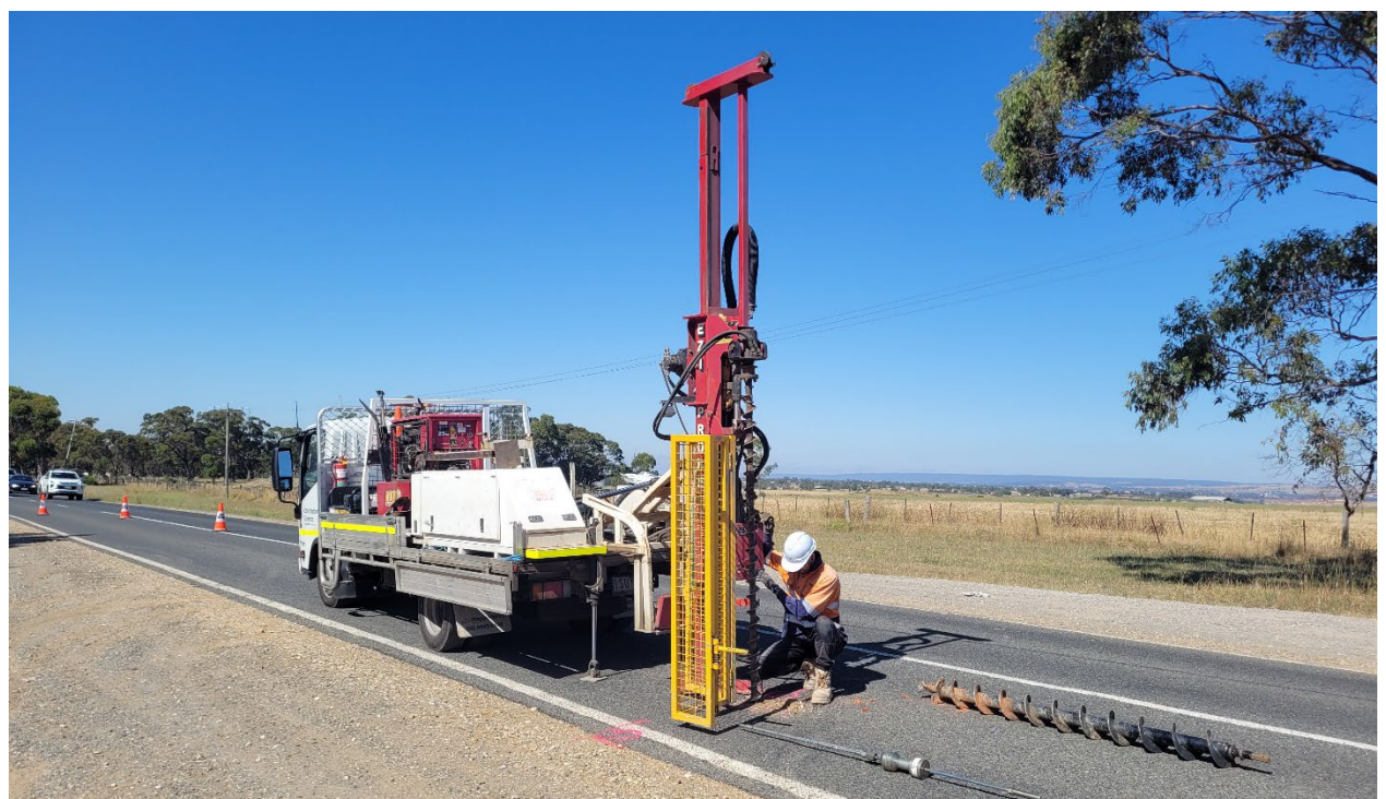
Image 20 – Drilling rig on BH06
