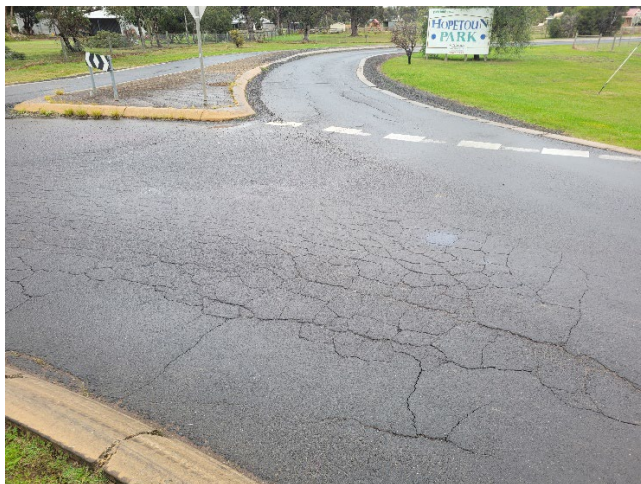
Image 5 – crocodile cracking, south west side of roundabout
