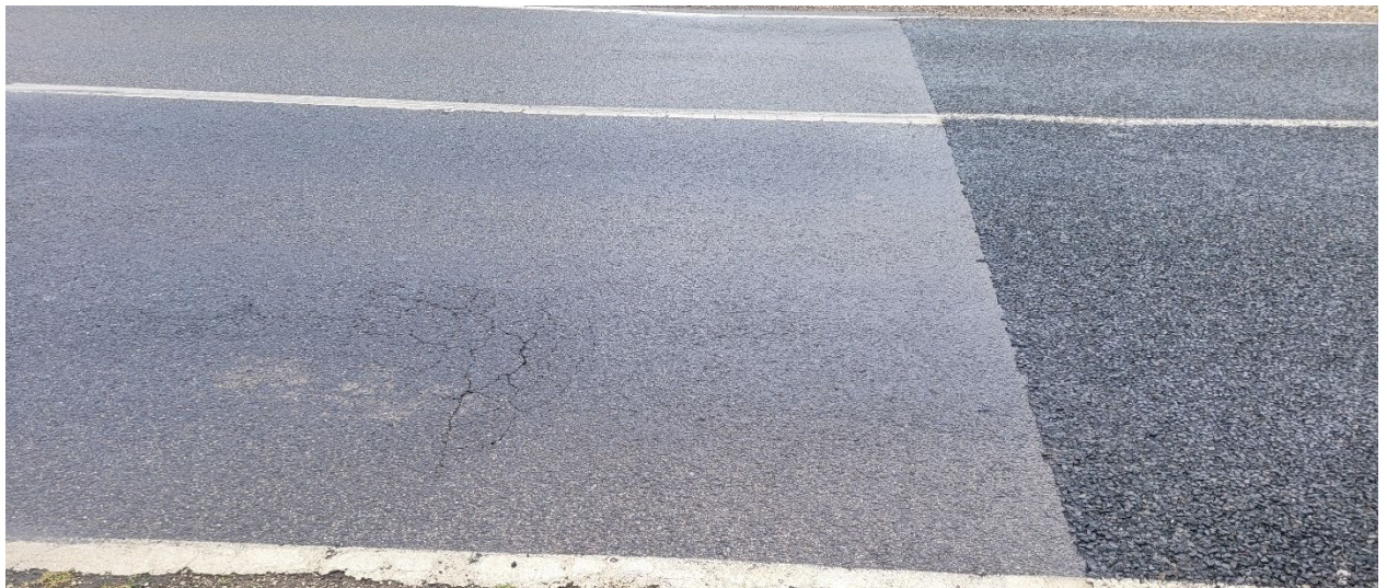
Image 10 – minor crocodile cracking in asphalt at north end and also showing the adjoining sprayed seal pavement
