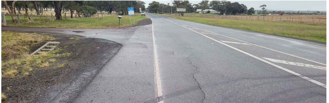
Image 9 – line cracking in asphalt at north end. The sprayed seal can be seen as the darker pavement to the south
