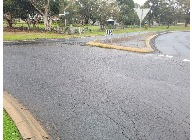
Image 6 – crocodile cracking, south side of roundabout
