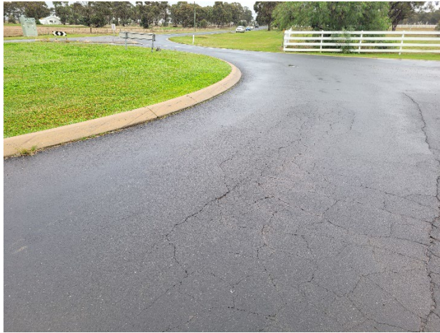
Image 3 – crocodile cracking, east side of roundabout, with some line cracking
