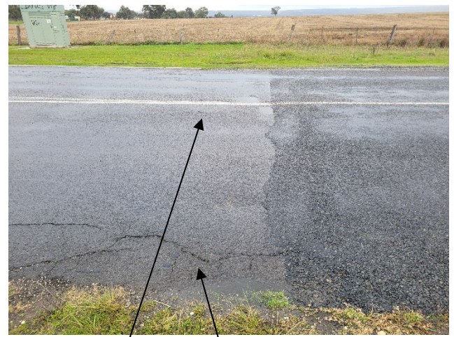
Image 8 – crocodile and edge cracking, southbound lane, north of roundabout where the asphalt abuts the sprayed seal
