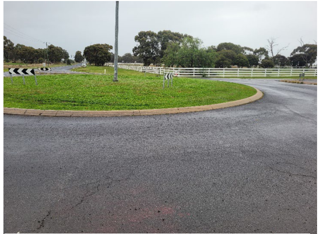
Image 4 – crocodile cracking, south side of roundabout looking north
