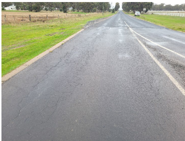
Image 7 – crocodile cracking, northbound lane immediately north of roundabout
