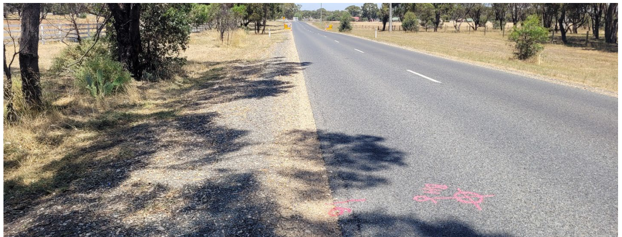
Image 15 – Edge of pavement near BH06 showing the overlay seal
