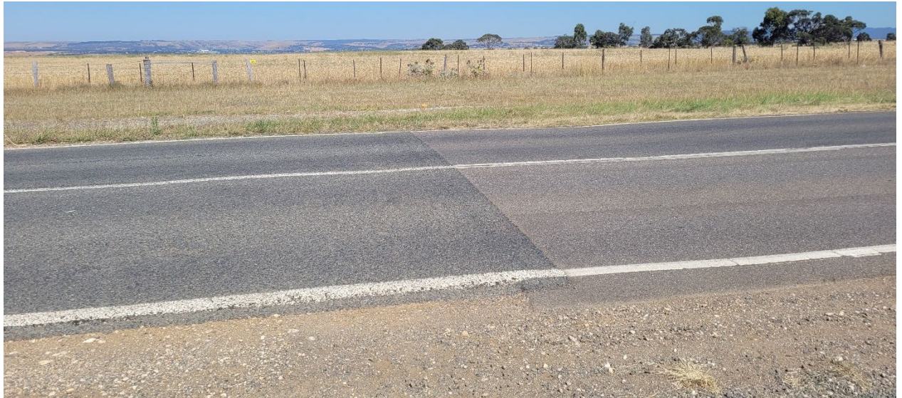
Image 14 – Change of pavement makeup about 100 m south of the Western Freeway, with the asphalt seal and cement treated crushed rock base on the right
