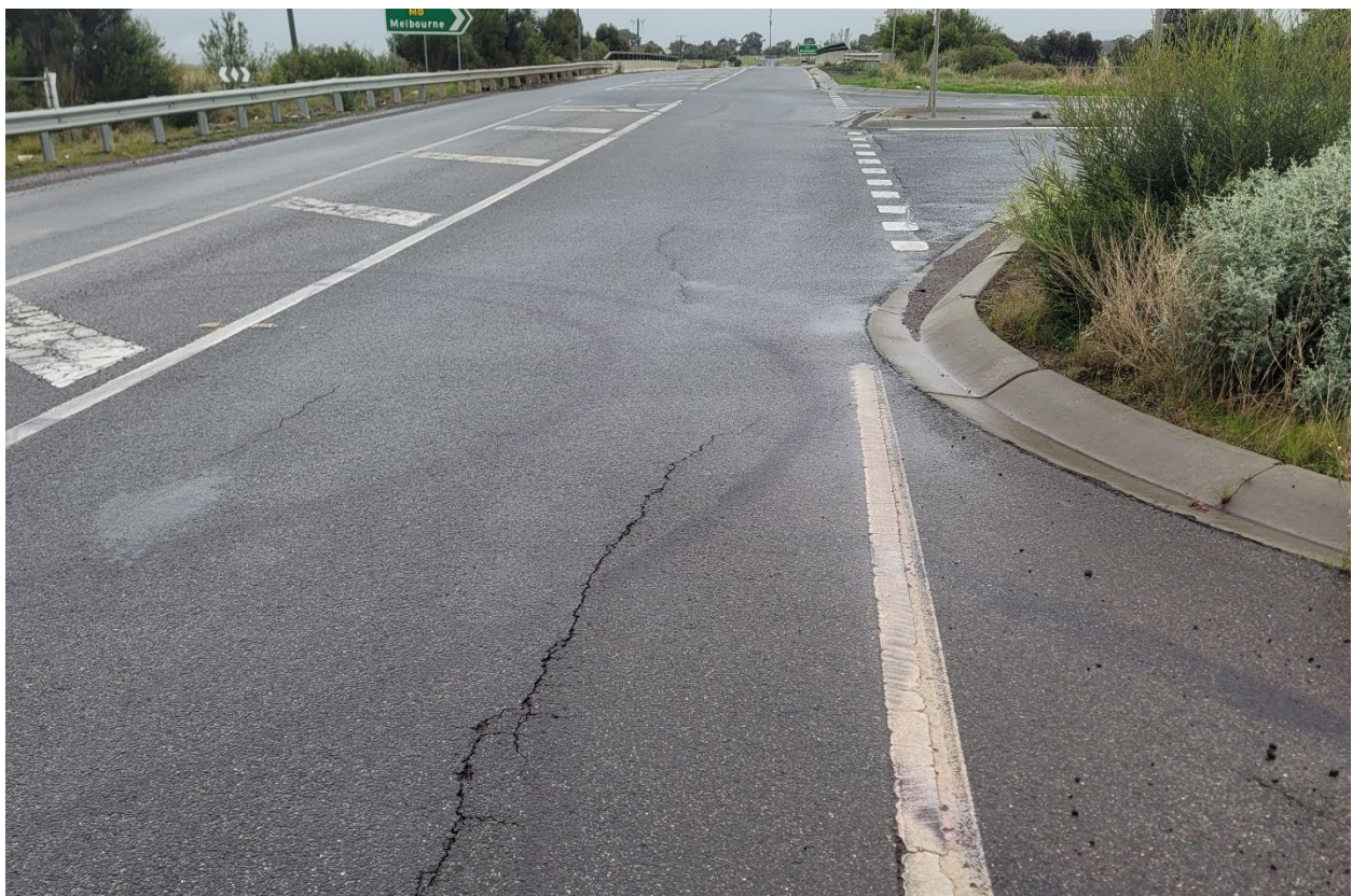
Image 11 – line cracking in north end asphalt, looking north
