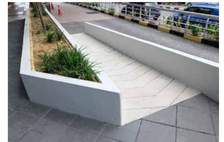
Off-form poured concrete
