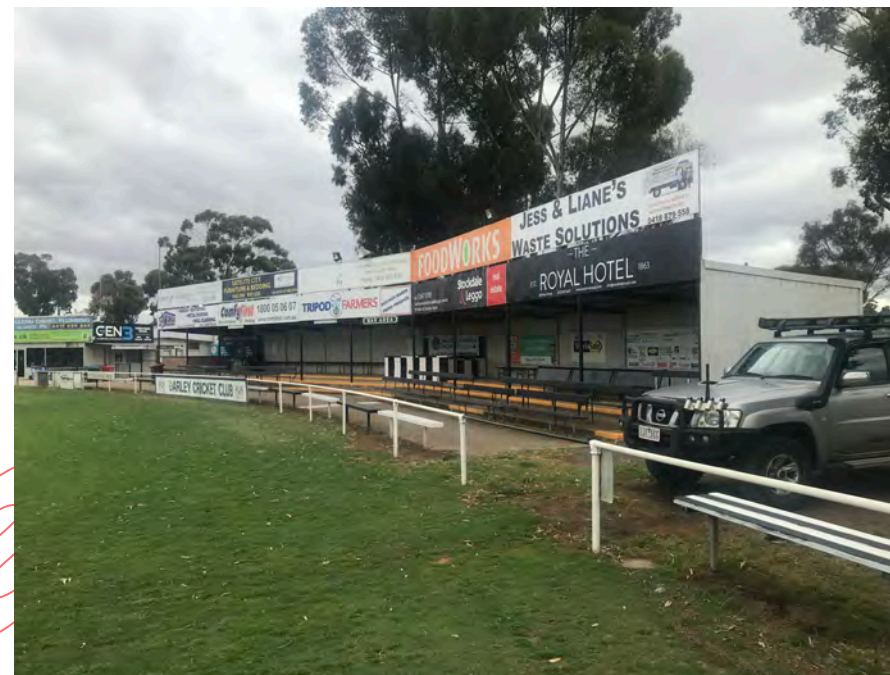
Figure 1. Grandstand on western side of Darley oval
