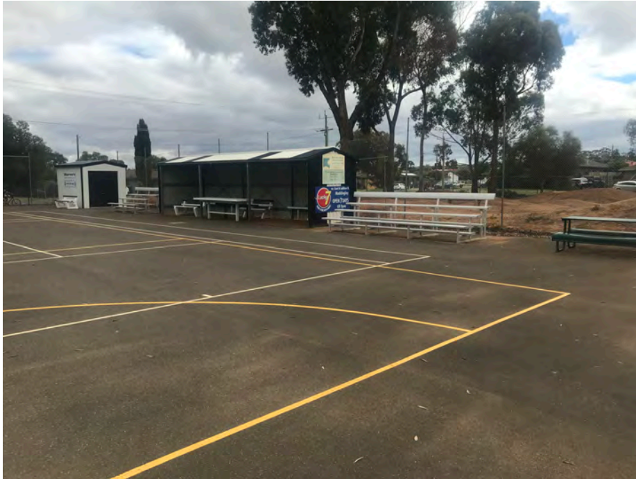
Figure 1. Netball/tennis courts (pre 2021 upgrade) and shelter
