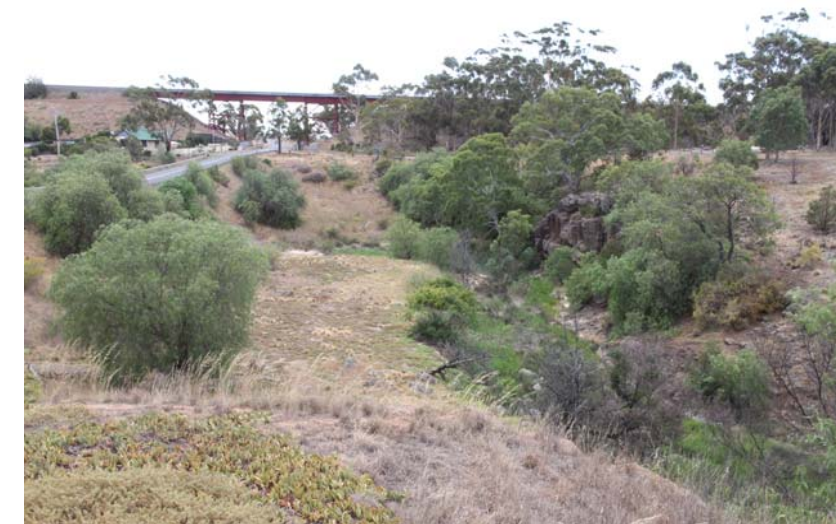
Photograph 3 Parwan Creek and railway bridge at southern boundary
