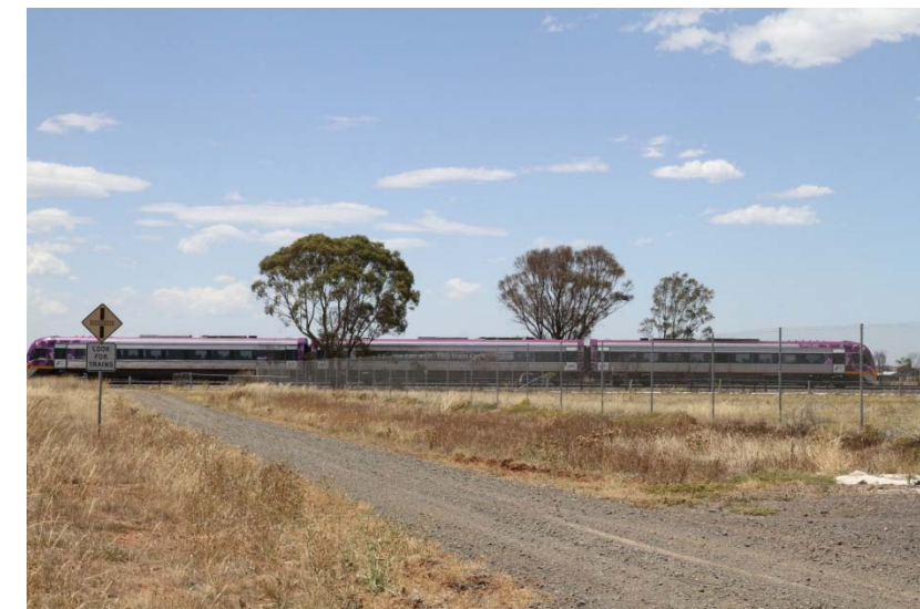
Photograph 8: Melbourne-Ballarat Railway Line at Albys Lane
