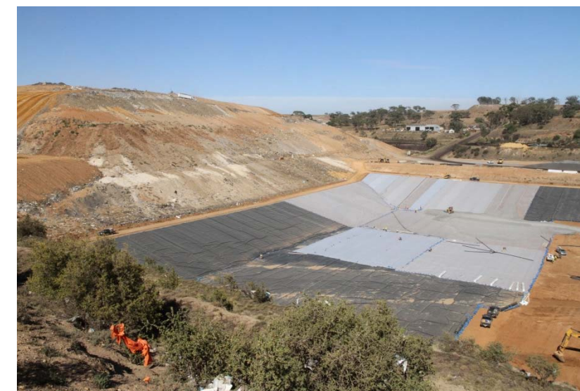
Photograph 4: Maddingley Brown Coal (MBC) active cell and Cell 2 under construction
